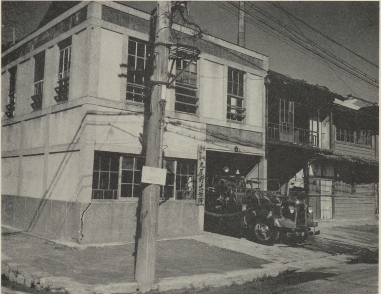
Photo 12. Maruo Substation. Partially damaged by atomic bomb, 9 August 1945.
